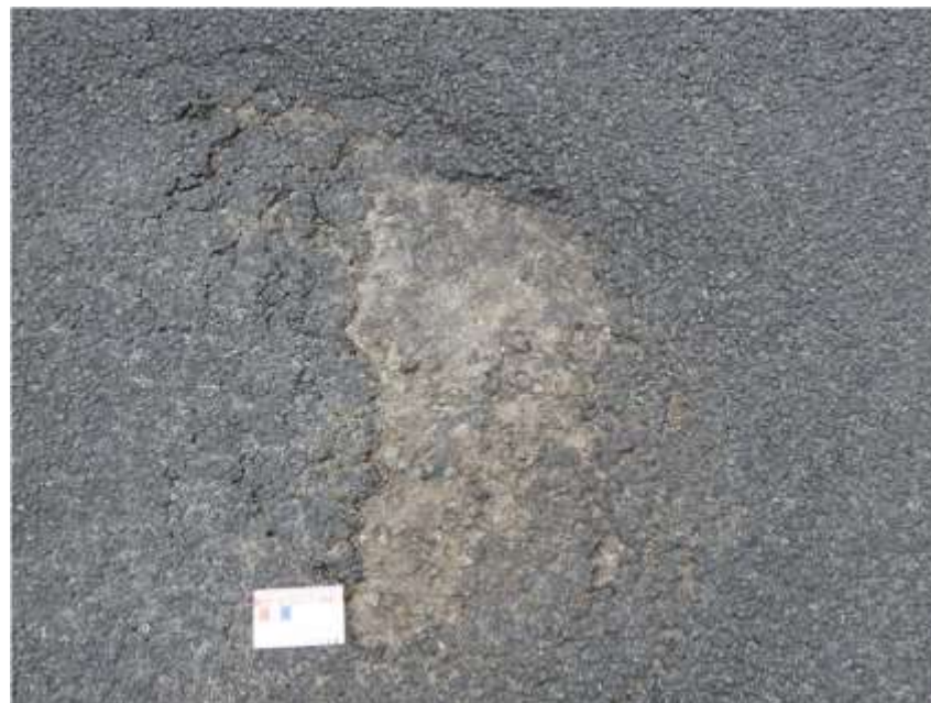
NOVACHIP(t=22mm)の損傷
